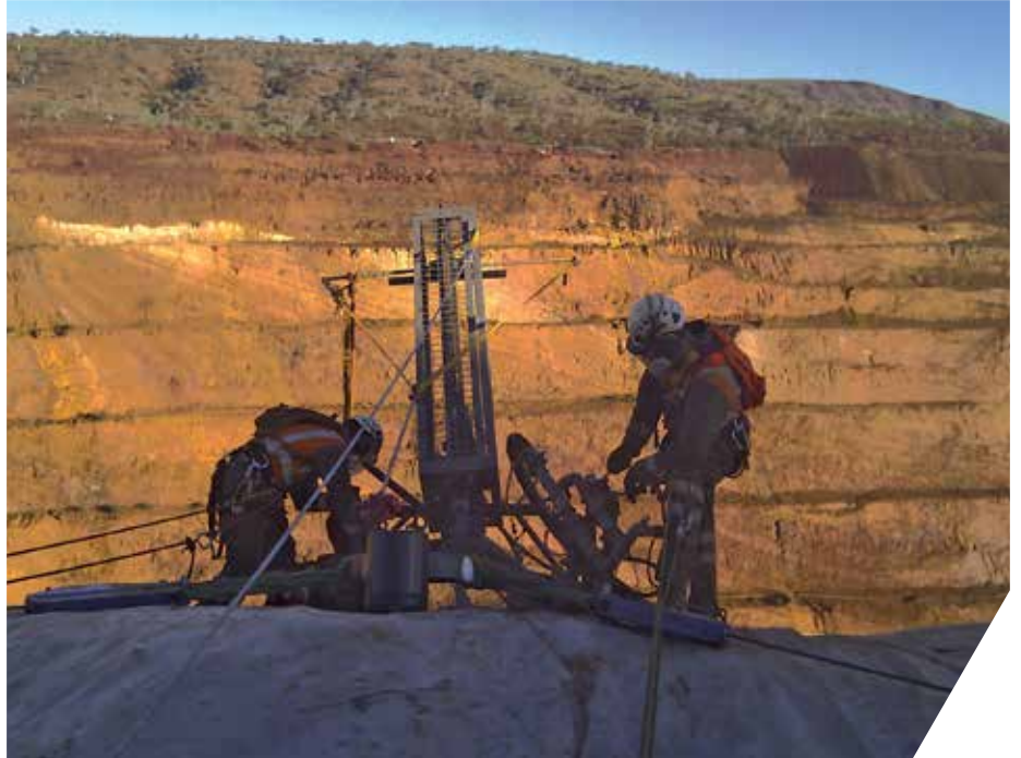
Above: SPIDER® net is made from a spiral steel rope and secures loose, blocky rocks, rock spurs, overhangs or unstable rock formations.
