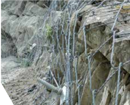
Above: SPIDER® net is made from a spiral steel rope and secures loose, blocky rocks, rock spurs, overhangs or unstable rock formations.
