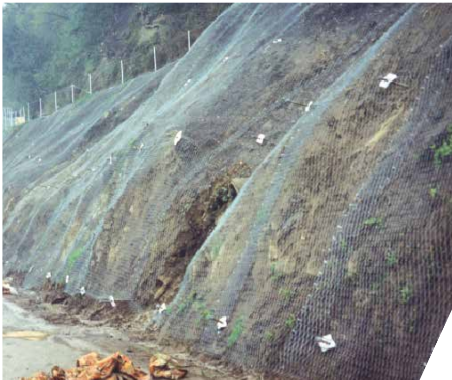
Fig. 40 (right): Protected slope in raw state
