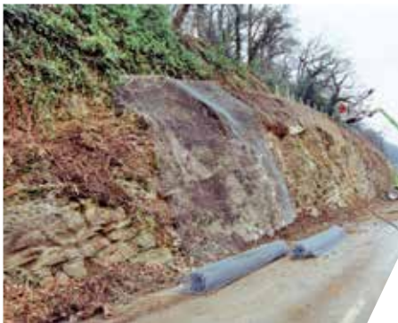
Fig. 39: Laying of the mesh sheets
