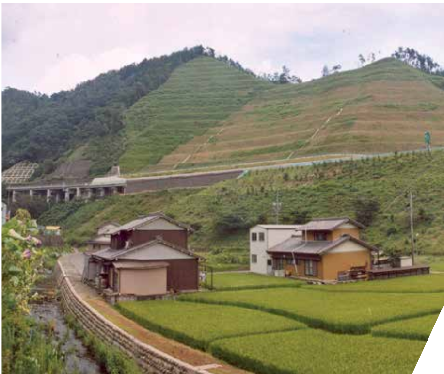
Fig. 6: Implemented project in Japan
