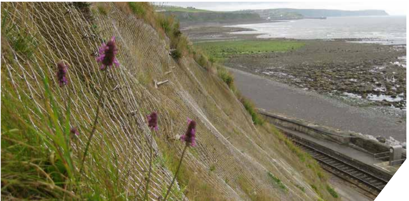
Fig. 48: Installation TECCO® G65/3 STAINLESS Parton Back of Rocks, United Kingdom
