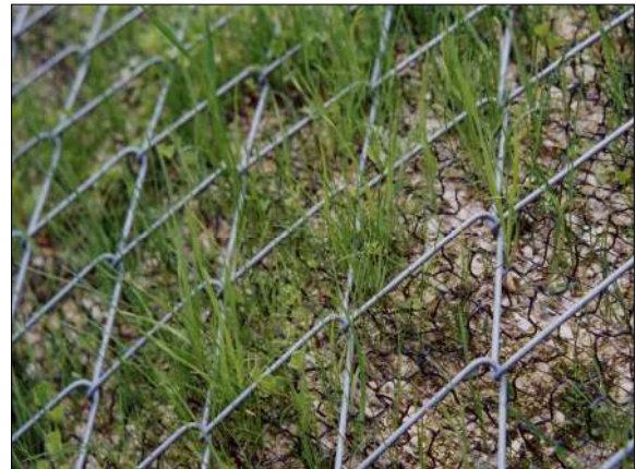
Figure 13. High-tensile steel wire mesh TECCO®
