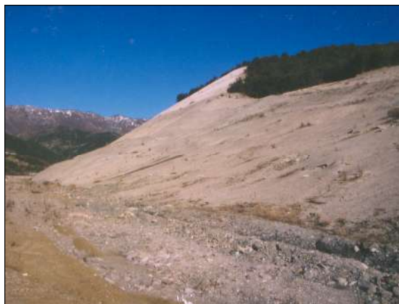
Figure 3. Shotcrete facing at location D
